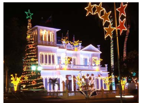
If you are unsure of what you are doing, contact a licensed electrician.
