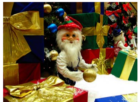
Don't cover transformers with presents or decorations. This is a common cause of fires at Christmas.
